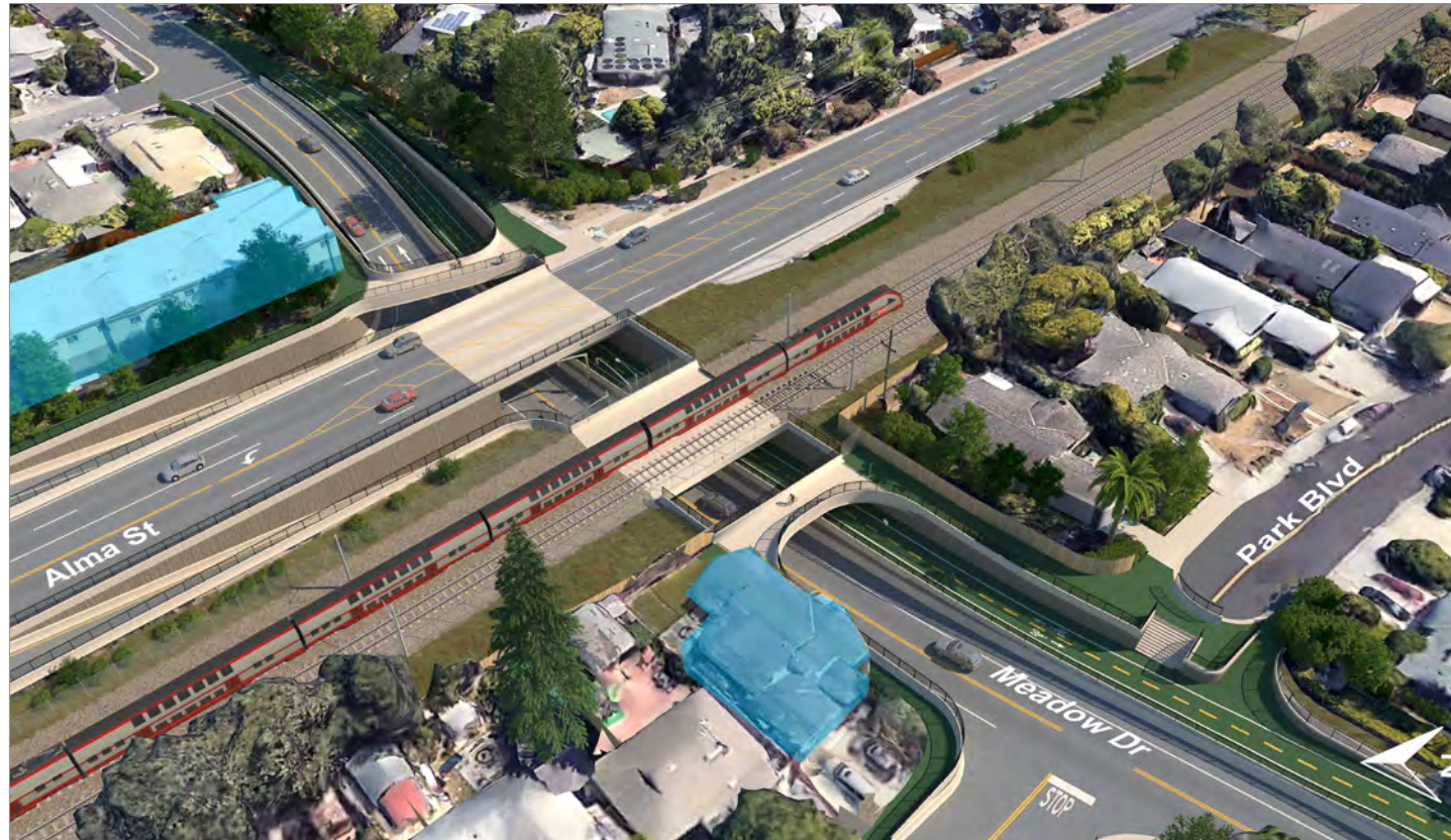
Meadow Drive Underpass Overview - Looking Southeast
