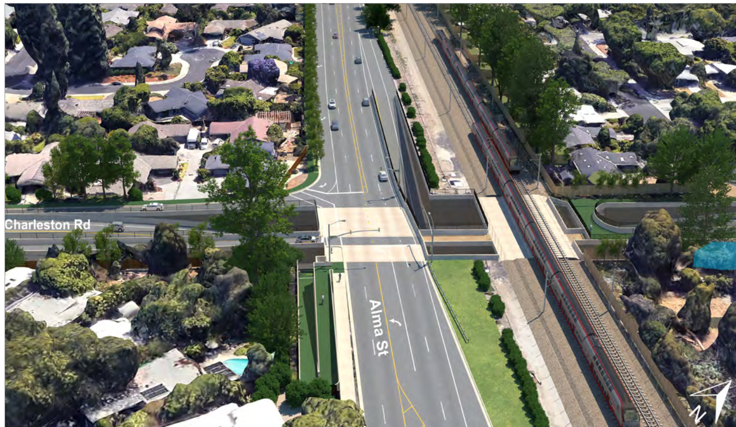
Charleston Road Underpass Overview - Looking South
