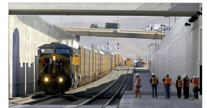
Trench in Reno, Nevada
