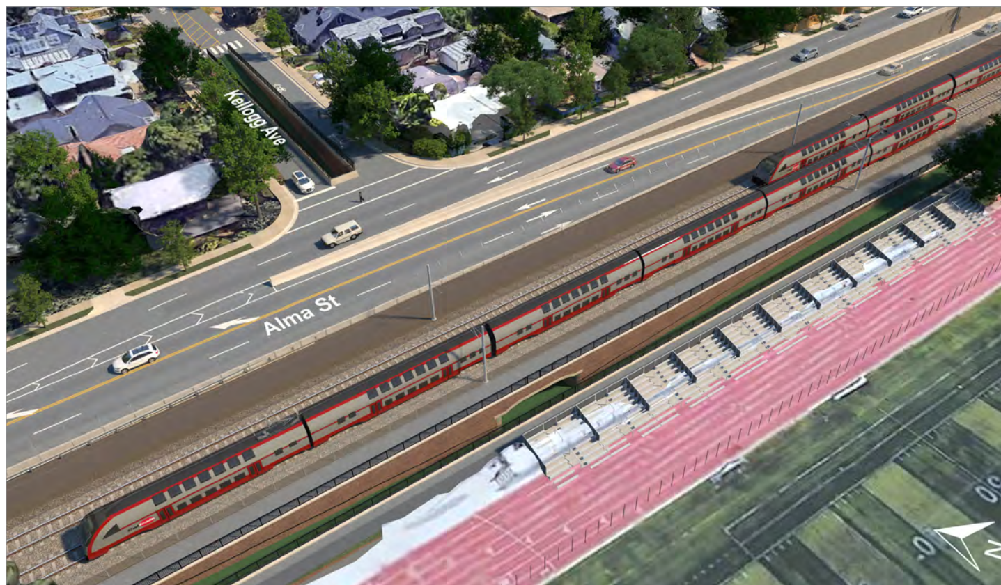
Kellogg Avenue Pedestrian/Bike Underpass - Looking Southeast
