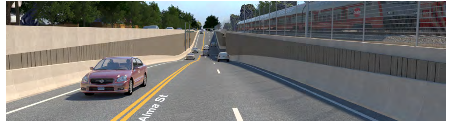
Lowered portion of Alma Street - Looking South Towards Churchill Avenue
