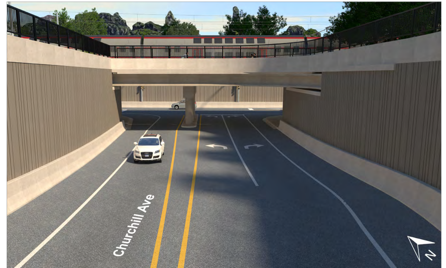
Churchill Avenue and lowered Alma Street Intersection with rail bridge and pedestrian/bike crossing - Looking East
