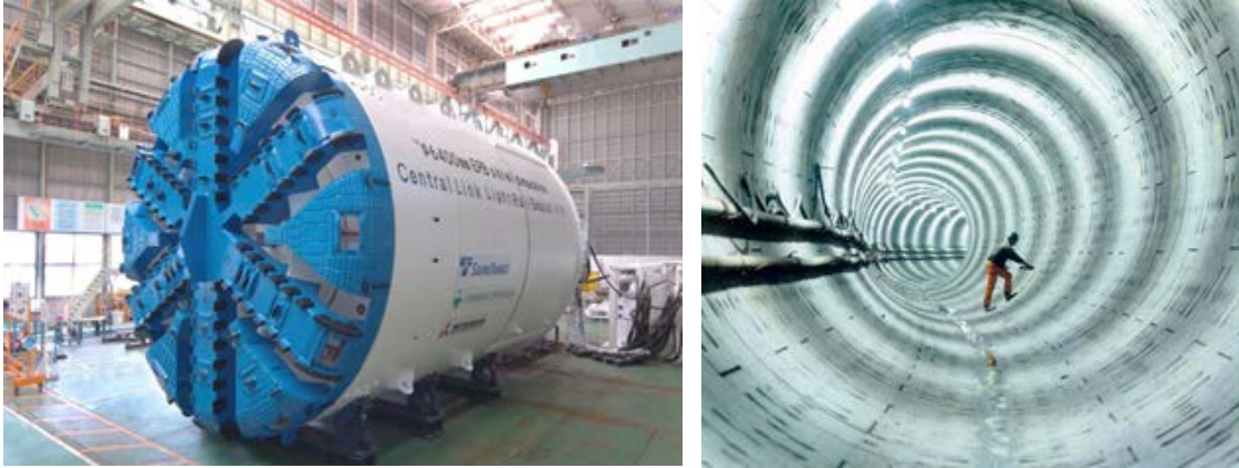
Figure 9: Tunnel Boring Machine (TBM) - Left; Completed Tunnel Lining - Right
