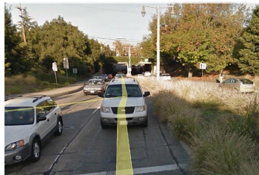
Figure 3-14: University Avenue Underpass, Looking East
