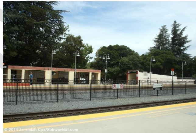
Figure 4-3: Palo Alto Caltrain Station
