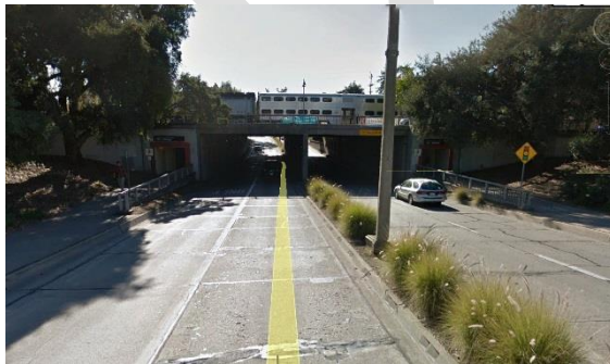
Figure 3-13: University Avenue Underpass, Looking West
