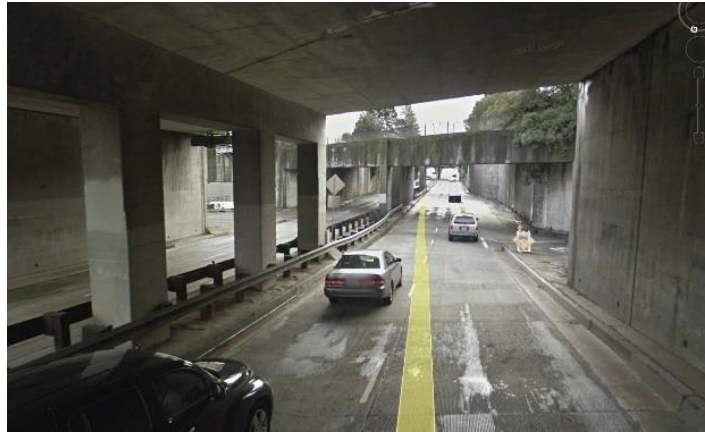
Figure 3-22: Oregon Expressway Underpass, Looking West
