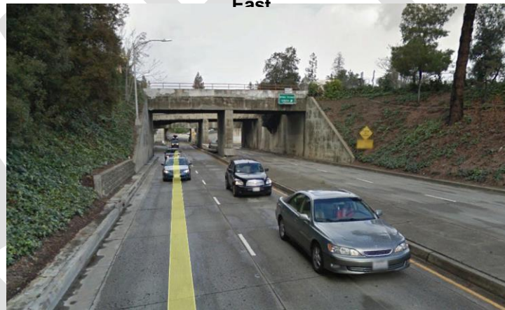
Figure 3-23: Oregon Expressway Underpass, Looking East
