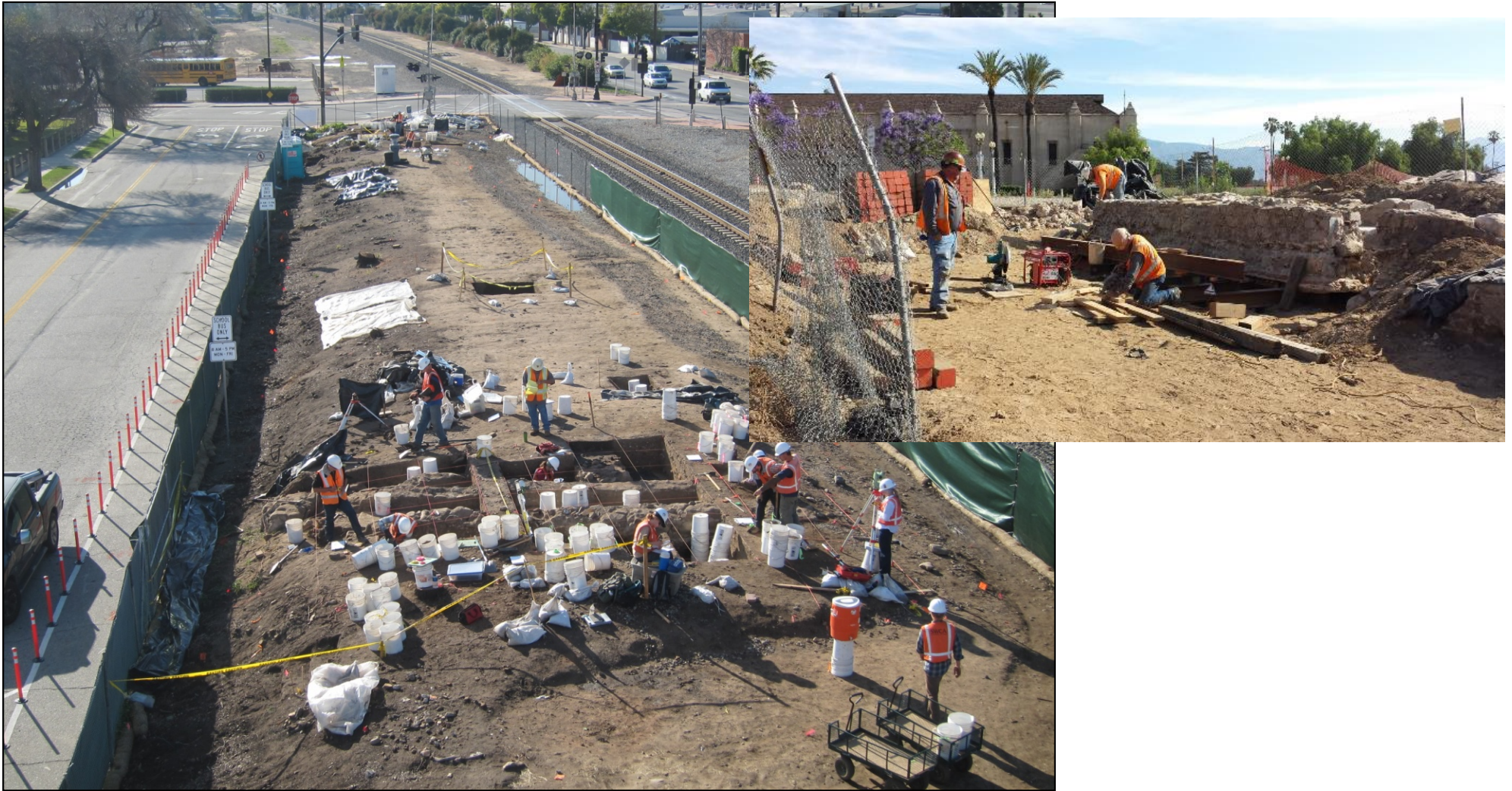
San Gabriel Trench Excavation Site
